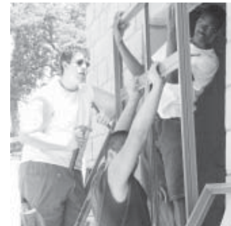
Installing windows in the new church building.
